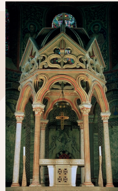
Monastery Maria Laach (Germany): the anterior two columns of the baldachin over the high altar made from lime deposit of the Eifel Aqueduct
