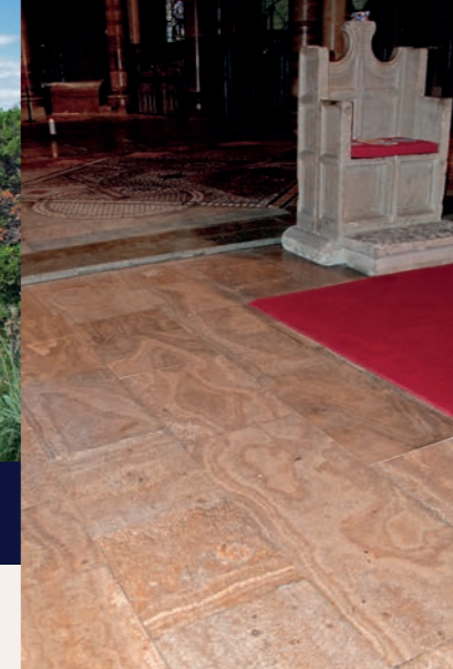
An export success of the middle ages: lime deposit from the Eifel Aqueduct as marble for the floor of the Bishop throne in the Canterbury Cathedral (England)
